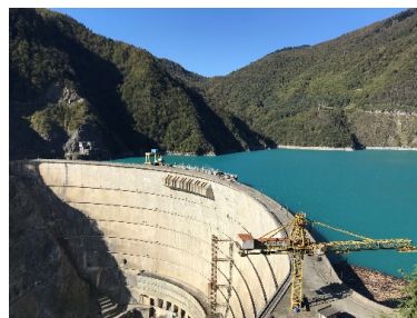
The 277 m high arch dam of the Enguri Dam in Georgia. © KIT-ACW
